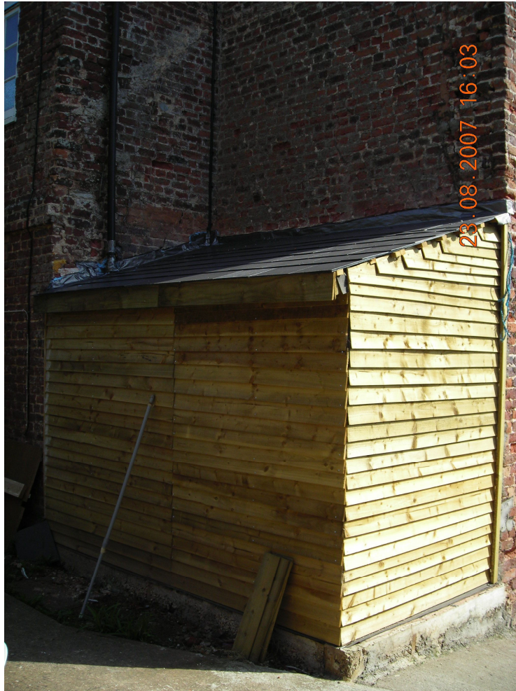
Extension at Pinbrook House, Chenyegate Lane
